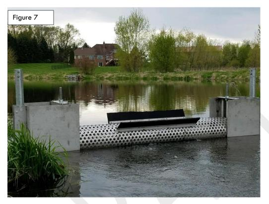
Action item 3.4.1- Install temporary PVC barrier at connecting channel and repair ferric chloride weir structure
