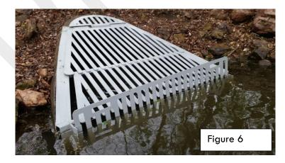
The barrier at the outlet of the desilt pond as installed in May of 2017. It is composed of a large drum wheel (16" diameter) that rotates with the flow of water. The drum is supported by a helical on each bank of the outlet and was installed to prevent carp from accessing the desilt pond as radio tags were documented in it in 2016.
