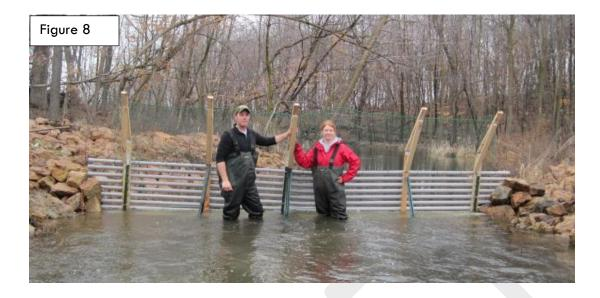
The final site that has been identified for a barrier is the existing ferric chloride injection site. The current structure is a weir wall with a cat walk above the top of weir to cross the stream, a series of rebar rods to act as trash racks, and a gate valve at the bottom of the weir wall. The rebar trash rack is in disrepair and is not capable of obstructing fish movement if the downstream water elevation is in equilibrium with the upstream water level.
